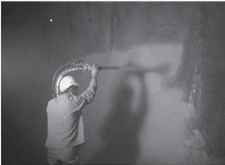
Figure 23. Manual application of Masterseal® 345 (Tunnel de Viret).
