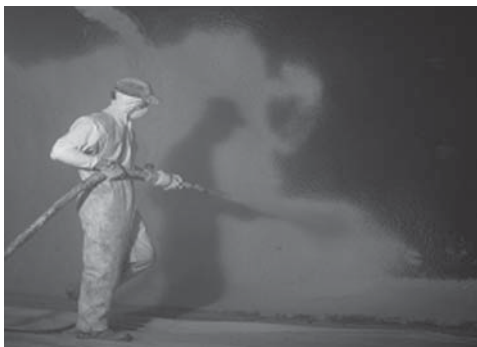
Figure 27. Manual spraying of the Masterseal® 345 membrane (Hirtenberger Ammunition Caverns).
