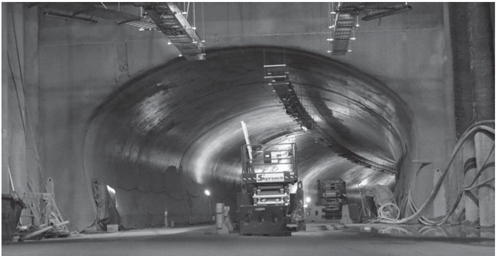
Figure 6. Shotcreted tunnel portals, north portal shown.
