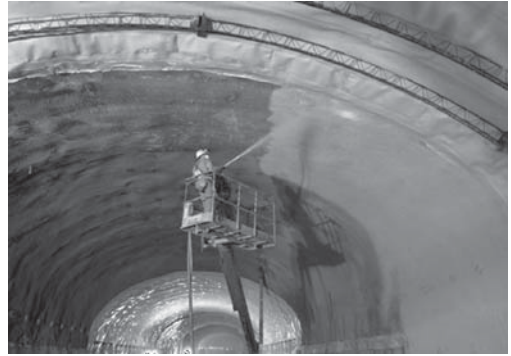
Figure 7. Fan niche waterproofing application.
