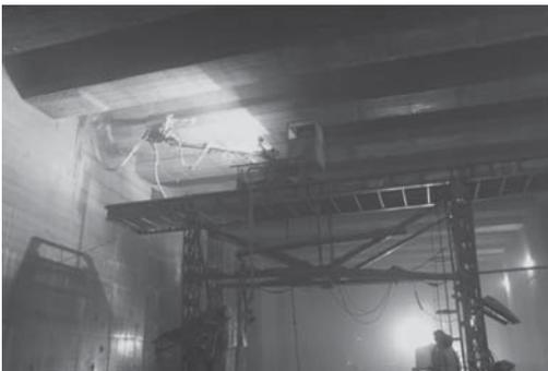
Figure 11. Shotcrete application at the hammer-head beams in the Tunnel Lainz, LT 23, Austrian railways (picture: Vogl).
