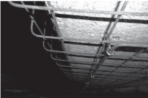
Figure 7. Example of mesh reinforcement together with anchorage for overhead application of shotcrete (picture: Ruzicka).
