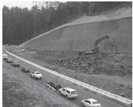
Figure 7. A simple well-sprayed gun finish, Mount Conjola NSW.
