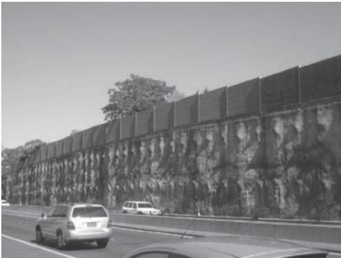
Figure 2. M2 motorway anchored wall—mesh ribbing is evident suggesting inadequate cover to reinforcement.
