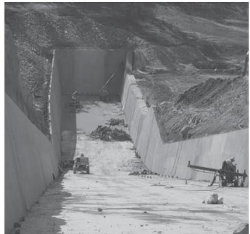
Figure 11. Shannon Creek Dam spillway and stilling basin.
