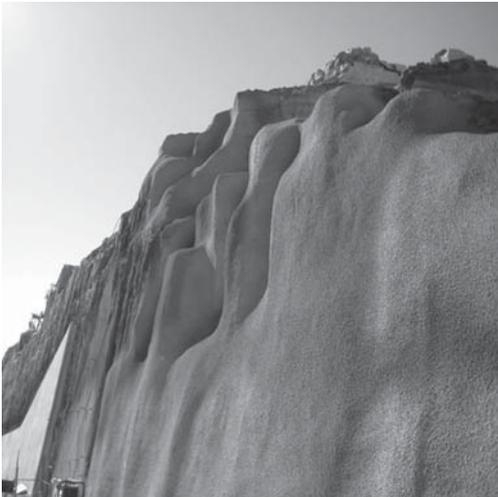
Figure 12. Off-the-gun or natural finish—Shannon Creek Dam, Grafton NSW—Embankment stabilisation.
