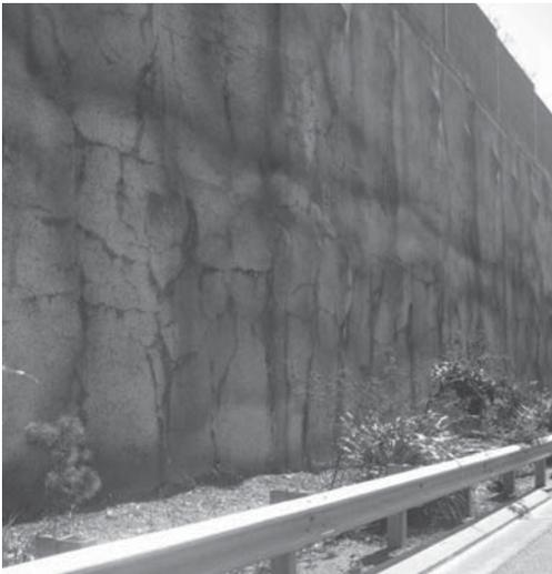
Figure 3. M2 motorway—another poorly staged and sprayed wall with excessive cracking.
