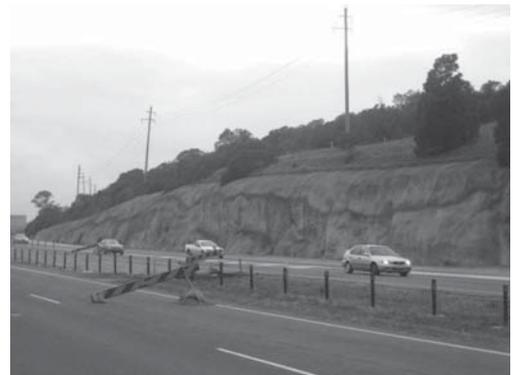
Figure 4. F6 freeway, Sydney—poor staging, poor spraying, overspray and excessive cracking.
