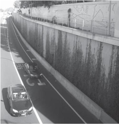
Figure 20. Shotcrete covered with pre-cast panels partly covered with creepers, Lane Cover Tunnel project, Sydney.
