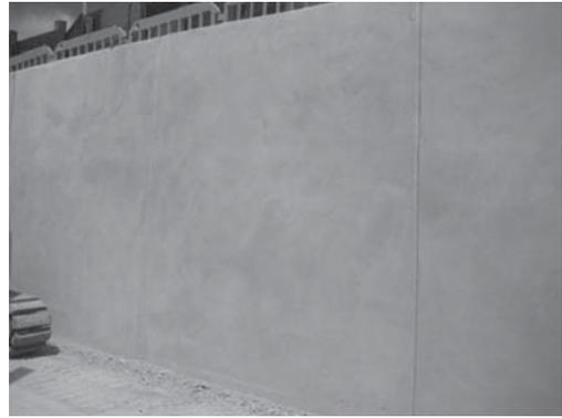
Figure 14. Wood float and sponge finish over Gun Finish along side pre-cast panels Cycle Way Clem 7 Tunnel Project Brisbane.
