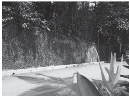
Figure 22. Creepers covering shotcrete wall in Singapore.
