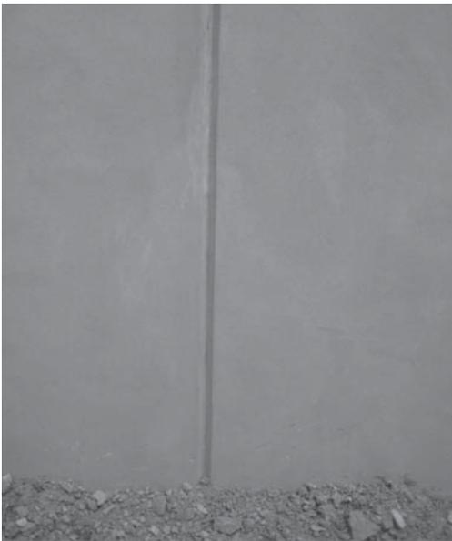
Figure 17. Dummy joint in shotcreted wall.
