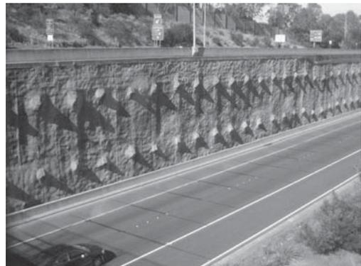
Figure 1. M2 anchored walls—poor staging, poor spraying, extensive cracking.
