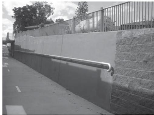
Figure 15. Wall completed with block work, WFS shotcrete and pre-cast panels, cycle way, Clem 7 tunnel project, Brisbane.
