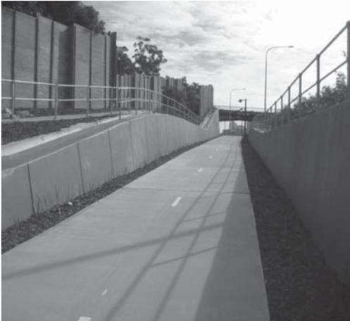
Figure 8. Finished walls with joints, LBBJV—Clem 7 for cycle ways (formerly North South Bypass Tunnel, Brisbane).
