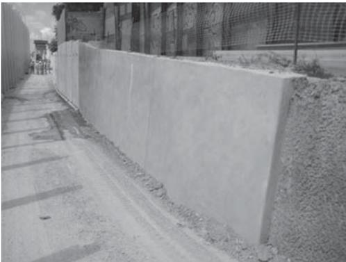
Figure 13. Wood float and sponge finish with dummy joints at 3 m intervals—cycle way, Clem 7 Brisbane.
