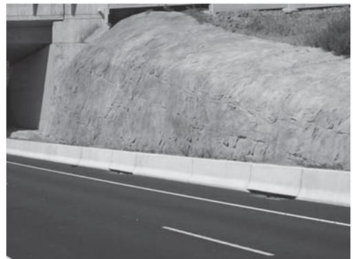
Figure 19. Simulated rock using shotcrete on side of M7 Freeway Sydney NSW.
