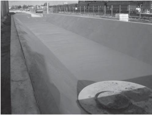
Figure 16. Steel trowel finish for an in-ground trough.
