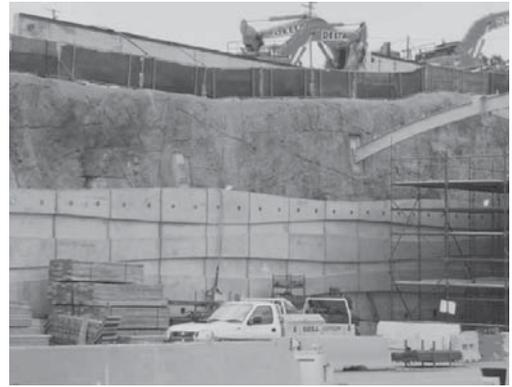
Figure 10. Simulated rock finish above pre-cast Clem 7 tunnel project, Brisbane.
